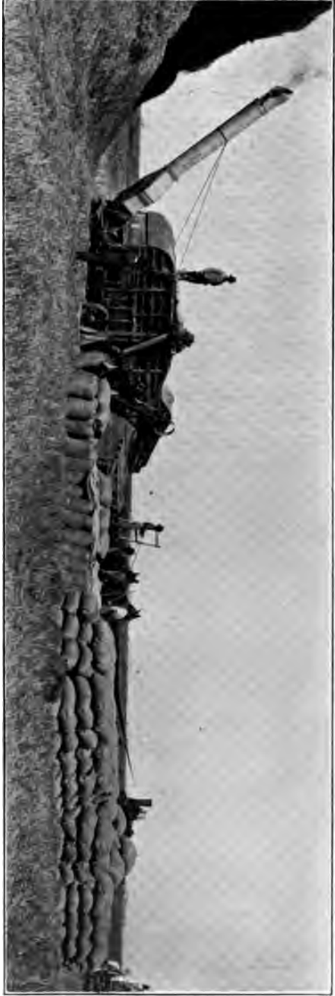
Photo from the Minneapolis Threshing Machine Co. THRESHING WHEAT IN MINNESOTA. Note the wheat in sacks ready for the market; the wagons with racks for hauling the bound grain to the thresher; and the engine which runs the thresher.
